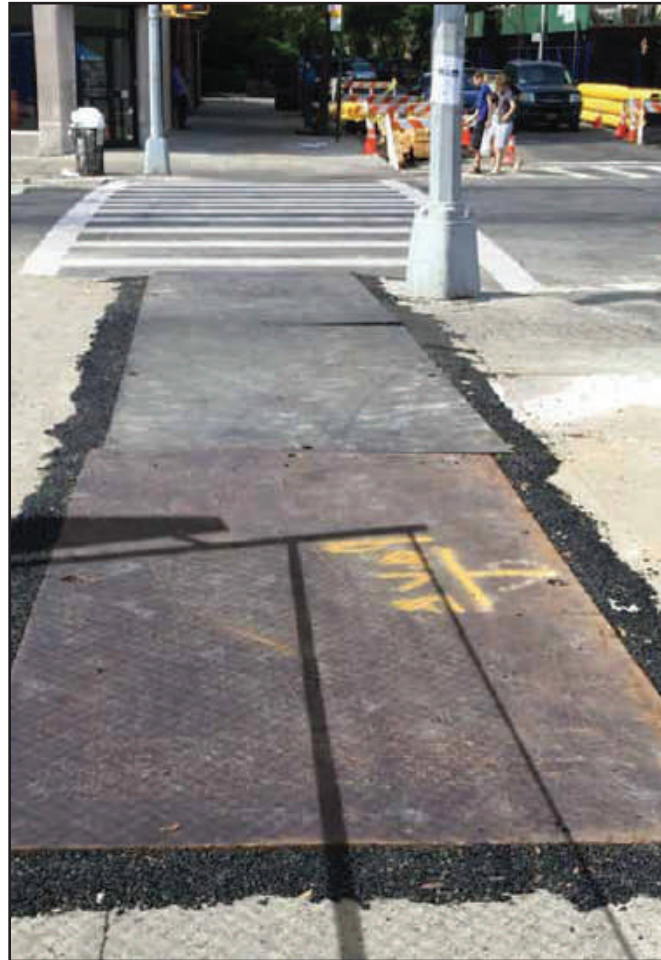
Steel Plates with Cold Patch
